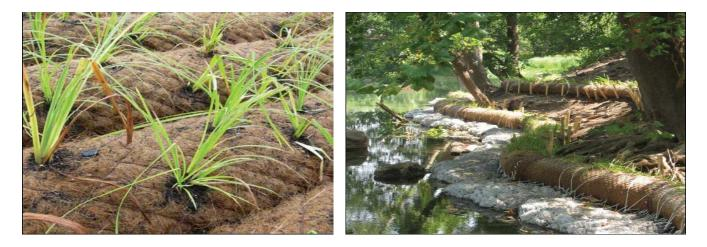
Typical Installation Method: Create a trench or seat to the dimensions of log and at the elevations specified. Lace logs with approved lacing material end to end to create a continuous length. Cross-lash rope front to back to prevent log from moving.
