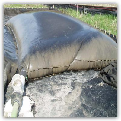
Hanes Geo Components dewatering filter bags are effective in collecting sediment during dewatering operations. Sediment-laden water is pumped into the bag.
